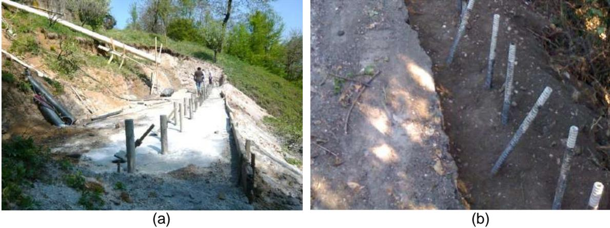
Figure 5. Examples of tie-back micropile wall in Vicenza Province: a landslide in Posina (a); a detail of micropiles easel with bar as reinforcement (b).
