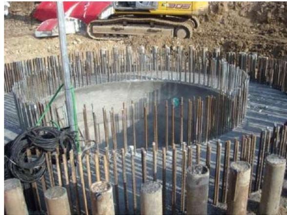
Figure 4. Realization of a structural well in Frana Fantoni (Recoaro).
